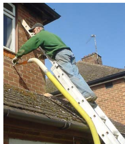
Figure 21.5. Cavity-wall insulation going in.
