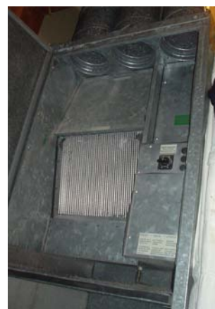
Figure E.11. The Heatkeeper's heat-exchanger.
