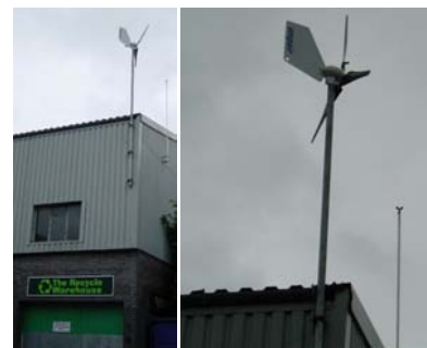
Figure B.9. An Ampair “600 W” micro-turbine. The average power generated by this micro-turbine in Leamington Spa is 0.037 kWh per day (1.5 W).
